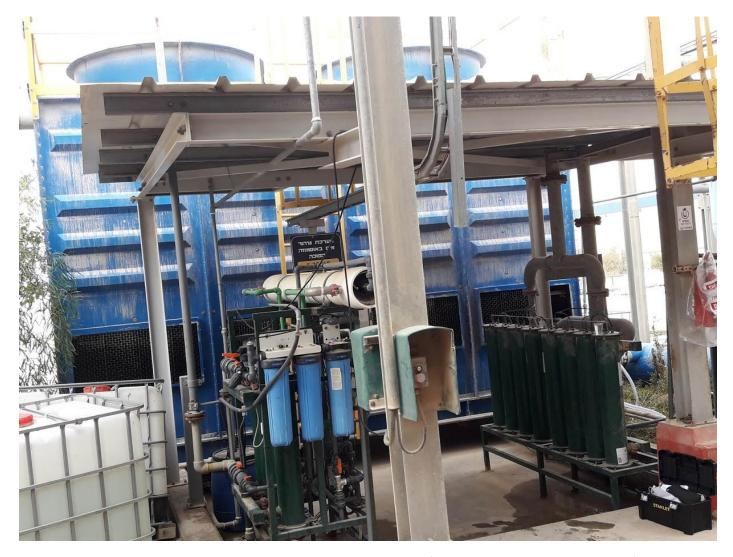
On the right side there is a UET-SR-CT unit, which circulates water from the basin to the UET unit, after which the treated water returns to the basin without any blow-down.
