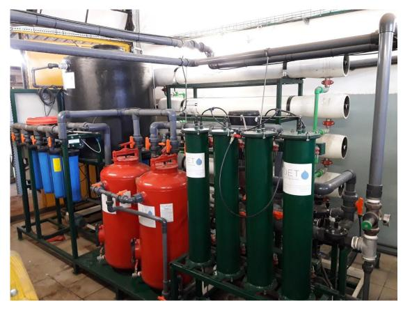
The RO system that removes minerals from the water using a UET-SR pre-RO system and an RO system that has a yield of 82% recovery
